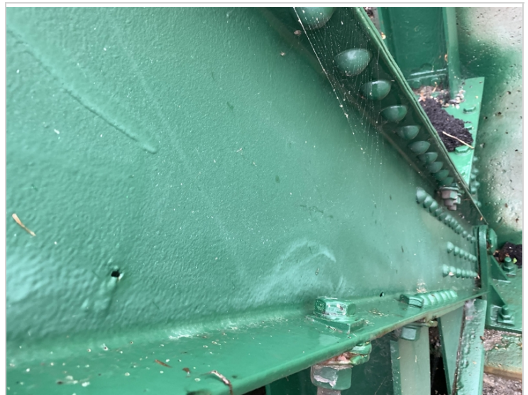
Diagonal 6 in truss 2 perforations
