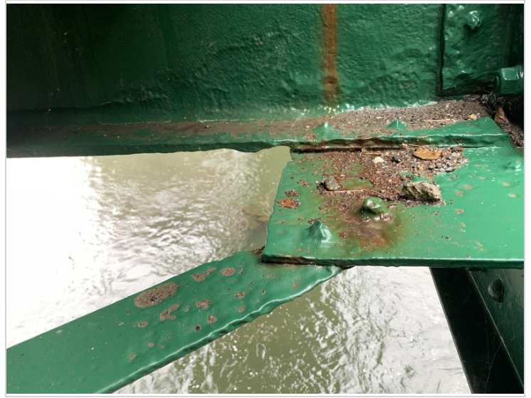
Section loss in floor beam 1 bottom flange
