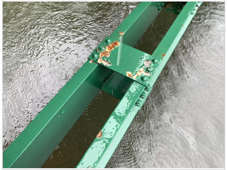
Hole in interior bottom chord of truss 2 between floor beam 4 and 5
