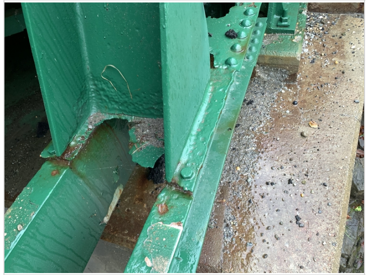
Section loss in exterior bottom chord at abutment 2
