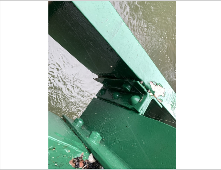
Typical section loss and heavy pitting along exterior bottom chords and rail post connections
