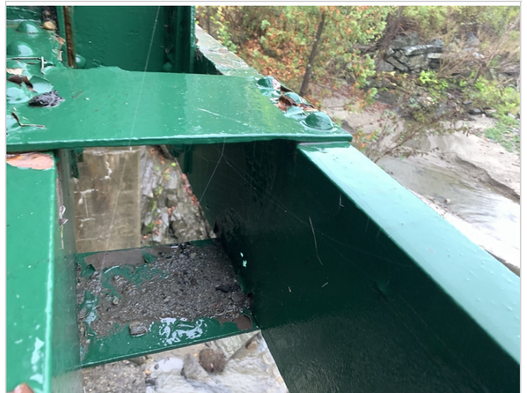
Perforation in exterior bottom chord near floor beam 5
