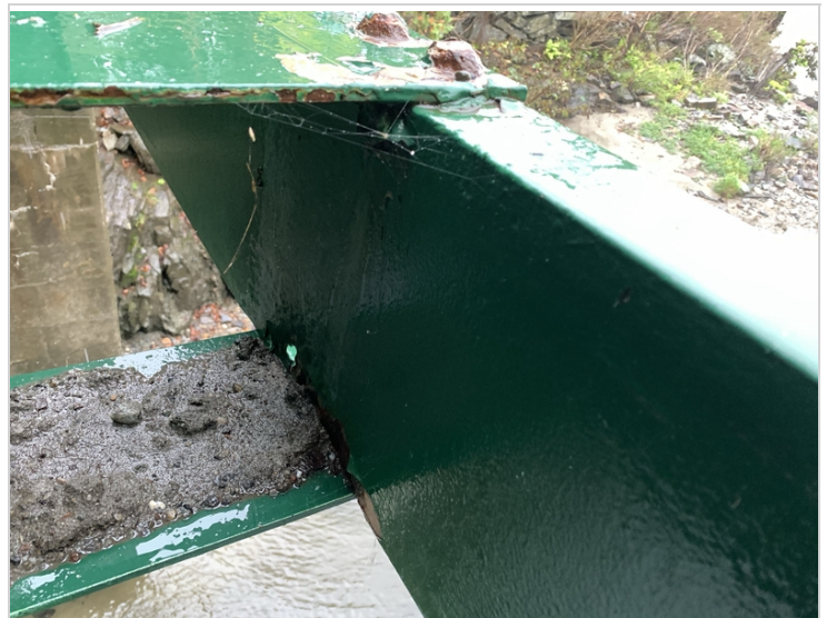
Hole in exterior bottom chord near floor beam 5
