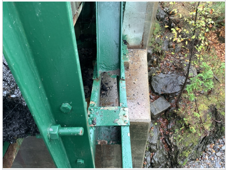
Distortion in bottom chord near abutment 2 truss 2
