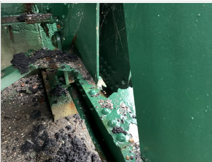
Section loss in interior bottom chord at abutment 2
