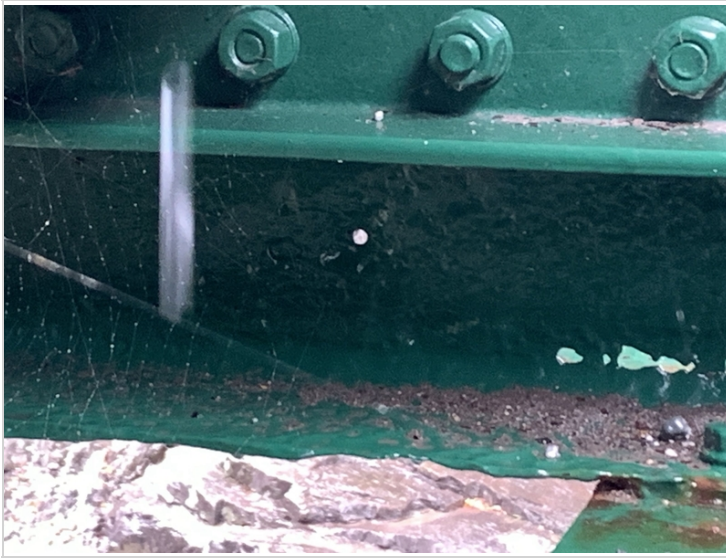
Holes in floor beam 4 truss 2
