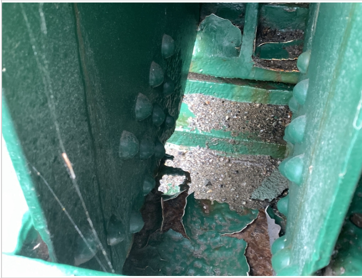
Heavy pitting in gusset plate 1 in truss 2 and perforations and section loss in stiffener plate
