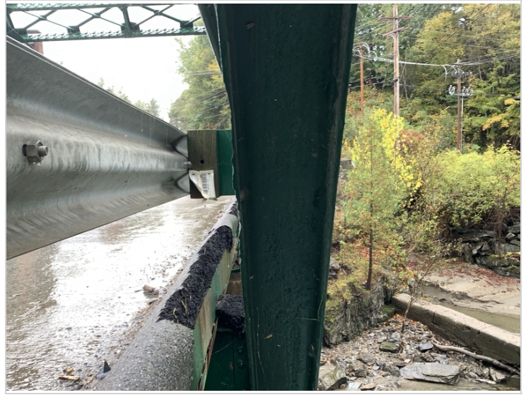
Section loss in diagonal truss 2
