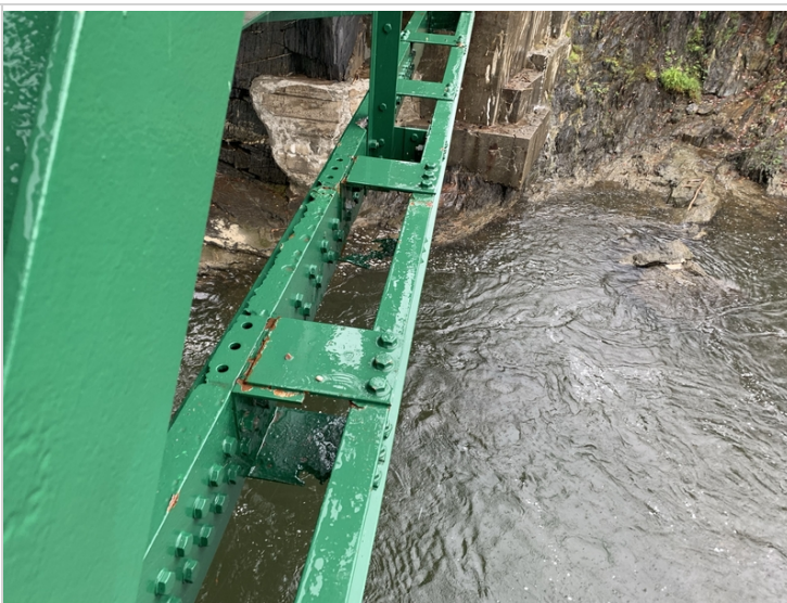
Bottom chord added steel plates and section loss truss 1 near abutment 2
