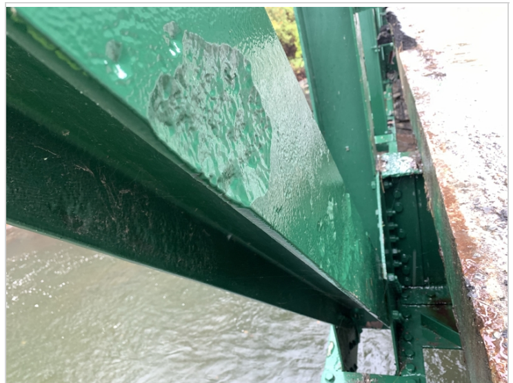
Previous pitting typical through out diagonals
