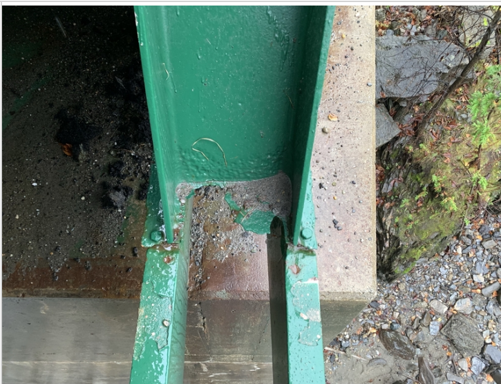
Distortion in bottom chord near abutment 2 truss 2
