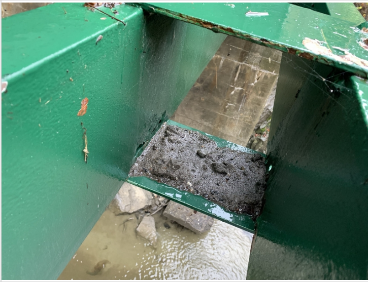
Hole in interior bottom chord near floor beam 5
