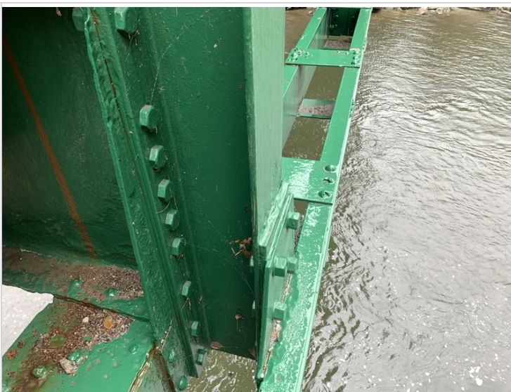
Previous pitting and section loss vertical 1 truss 2
