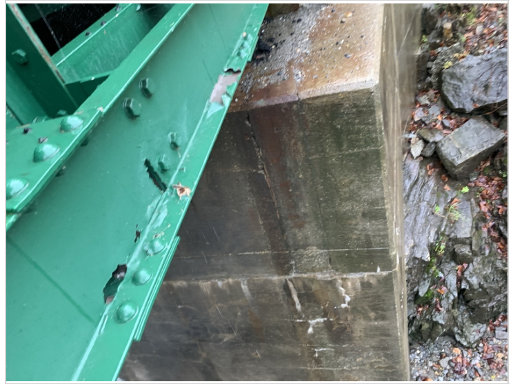
Holes in exterior bottom chord near rail post 6 truss 2
