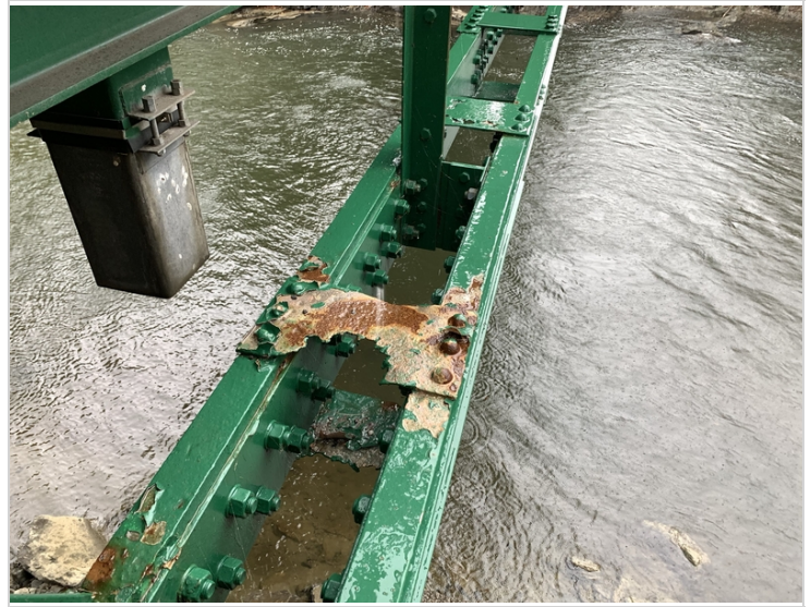
Bottom chord added steel plates and section loss truss 1 near abutment 2
