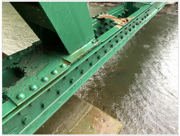
Bottom chord section loss near abutment 2 upstream end
