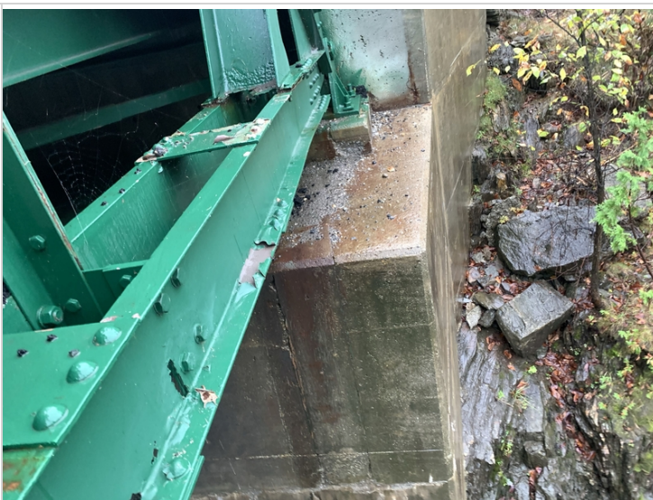
Distortion in bottom chord near abutment 2 truss 2
