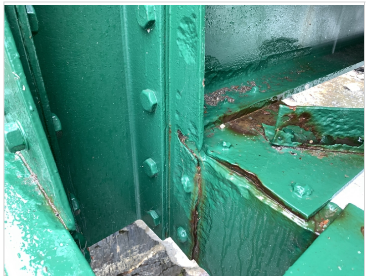
Perforation in flange of vertical 3 in truss 2
