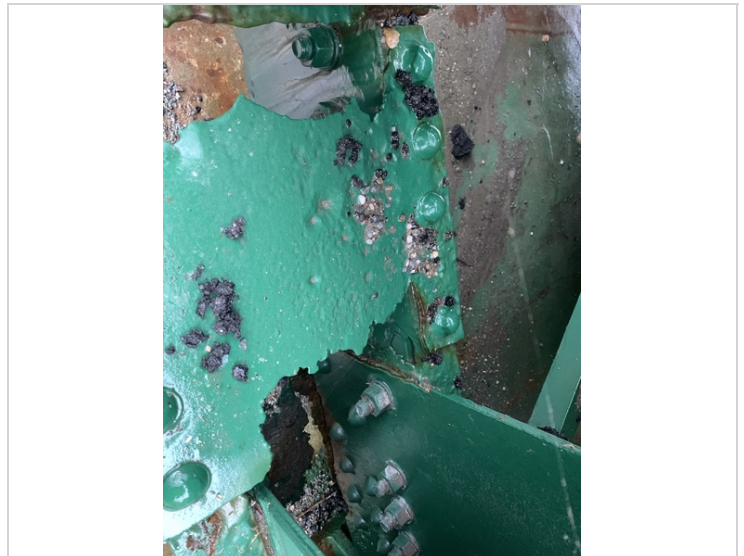
Hole in bottom chord with stiffener in place at abutment 2 gusset plate 7
