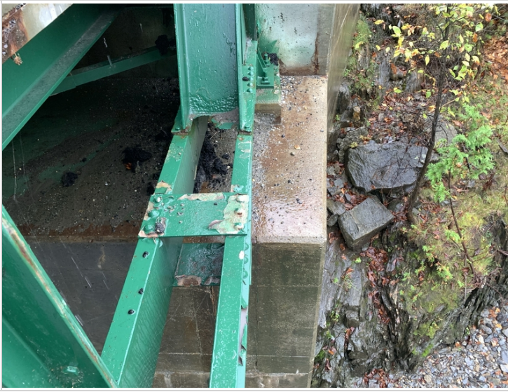
Distortion in bottom chord near abutment 2 truss 2
