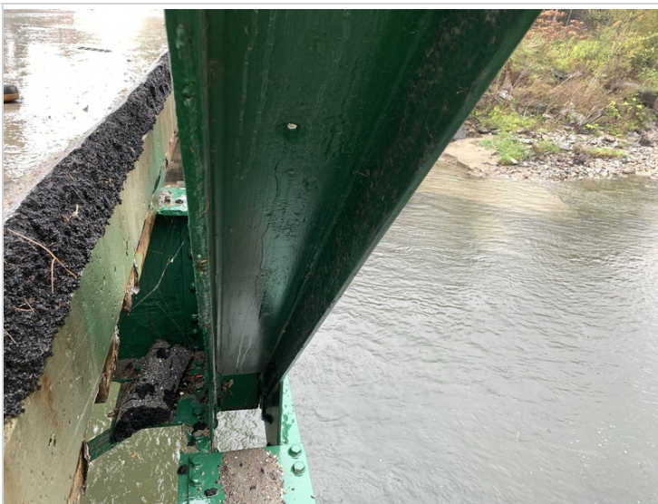
Hole in diagonal web truss 2
