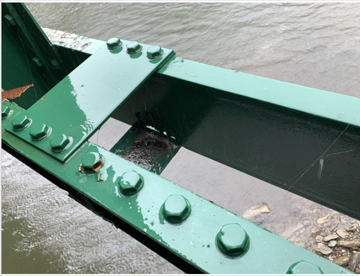
Perforations bottom chord between floor beam 4 and 5
